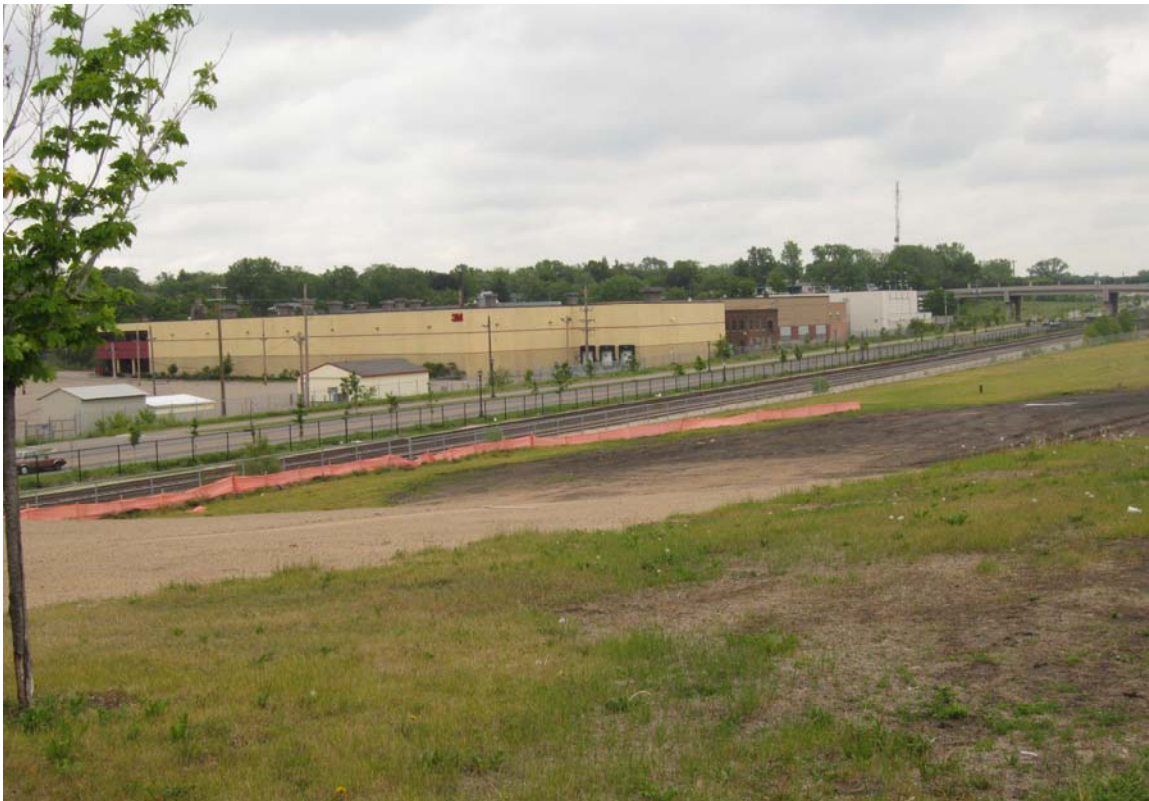
Figure 5. Building 47 site and Building 99 complex, looking northeast from Forest Street
