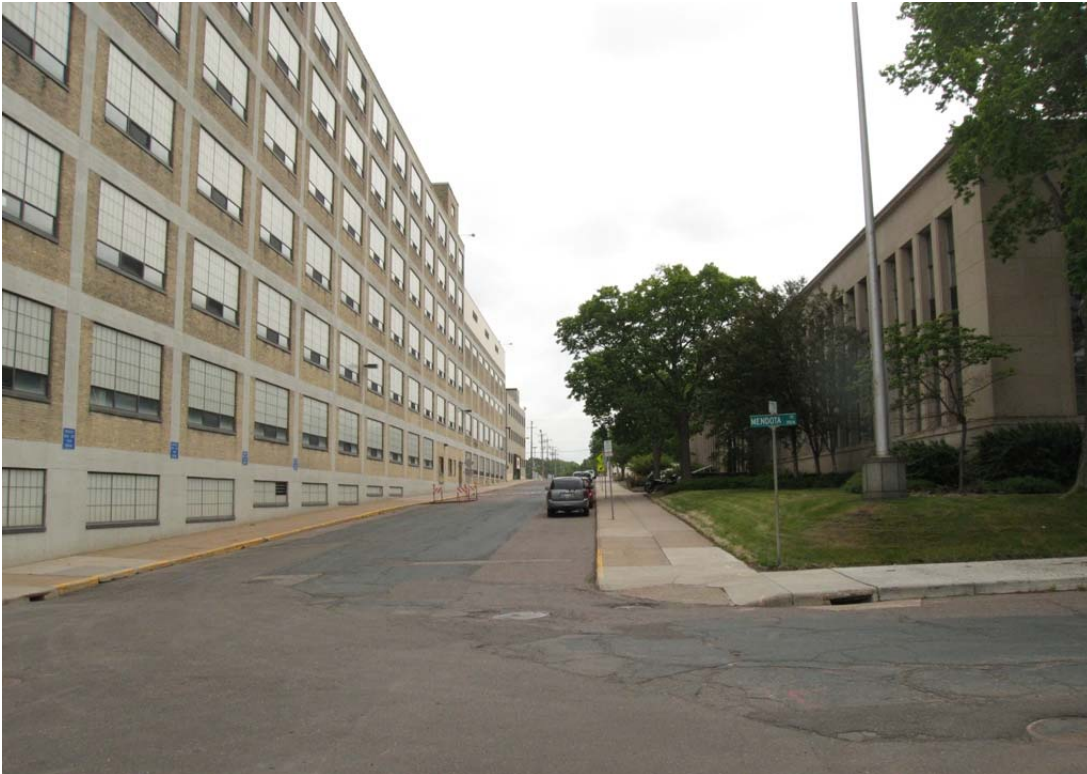
Figure 1. Buildings 20 and 21 and Bush Avenue, looking east
