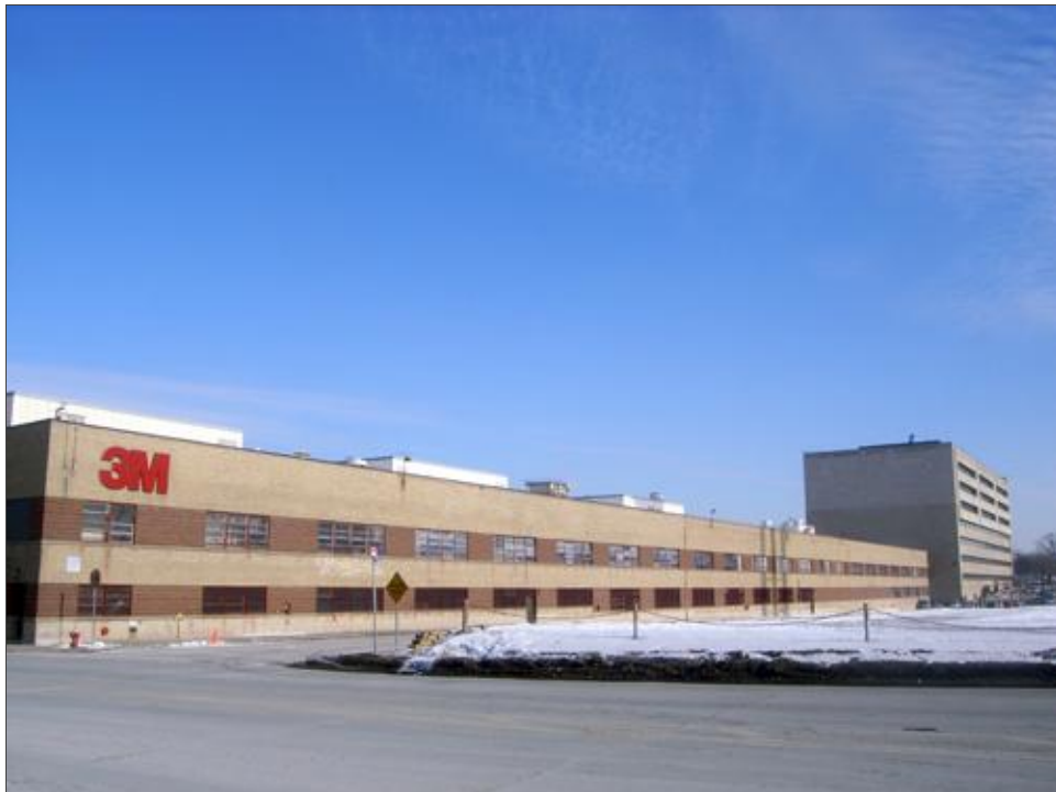
FIGURE 14. BUILDING 24, SOUTH ELEVATION, FACING NORTHEAST
