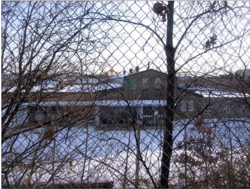
FIGURE 24. BUILDING 83, NORTH ELEVATION, FACING SOUTH
