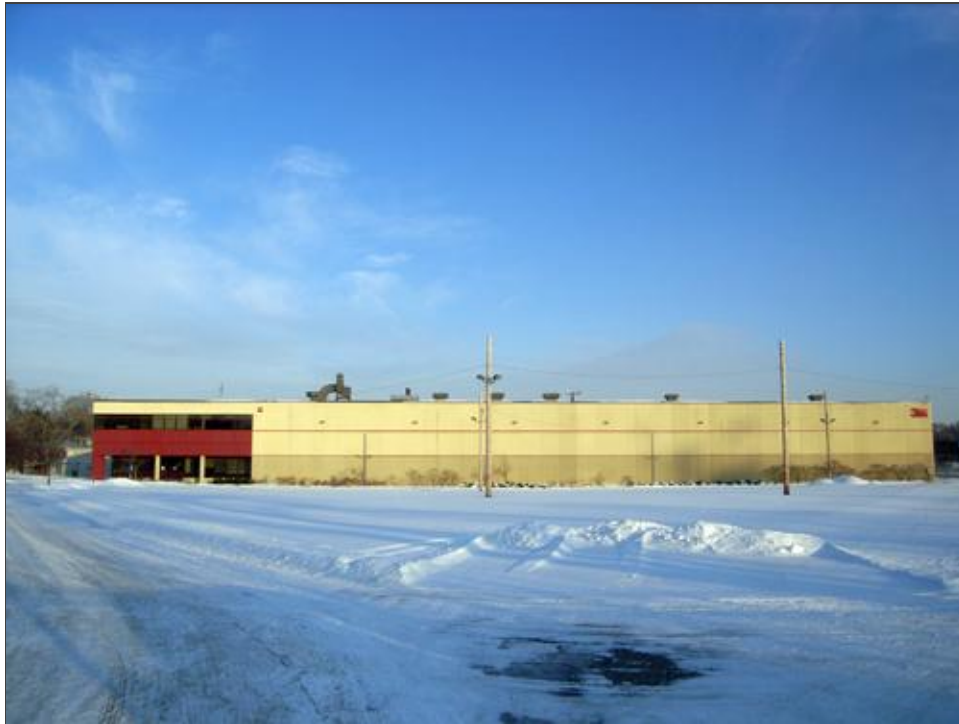
FIGURE 29. BUILDING 99, FAÇADE, FACING EAST
