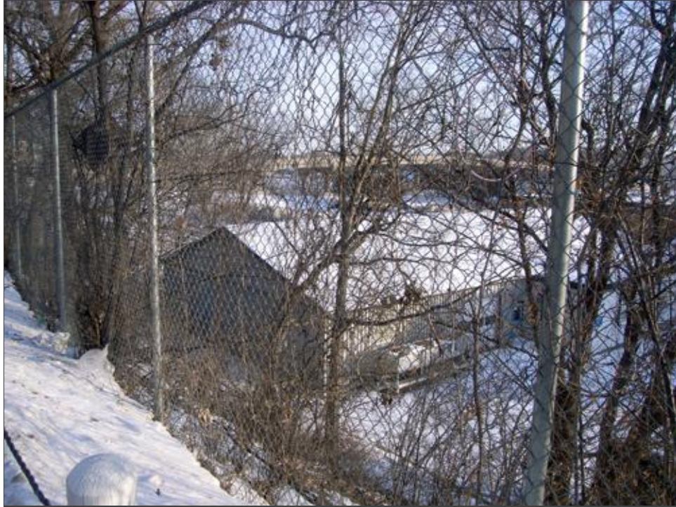
FIGURE 25. BUILDING 95, FAÇADE AND NORTH ELEVATION, FACING SOUTHEAST
