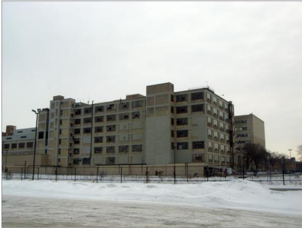
FIGURE 10. BUILDING 20, NORTH ELEVATION, FACING SOUTHEAST
