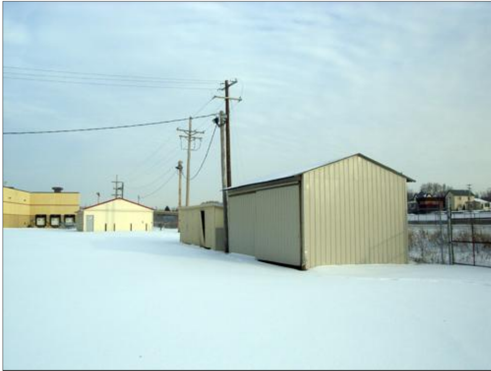
FIGURE 22. BUILDING 85, FAÇADE AND WEST ELEVATION, FACING EAST
