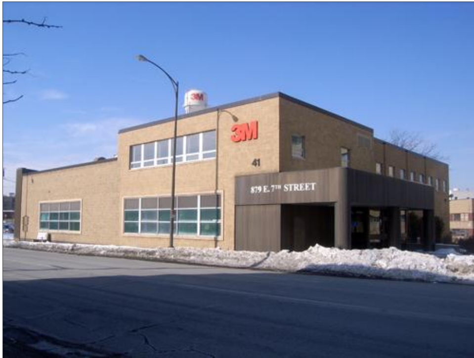
FIGURE 19. BUILDING 41, FAÇADE, FACING NORTHWEST
