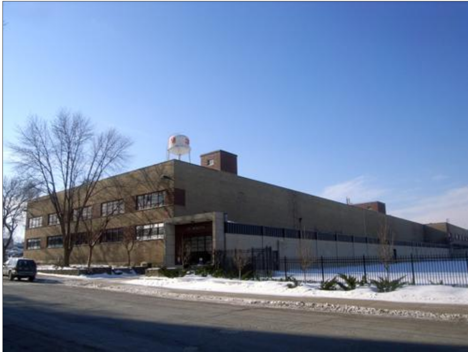
FIGURE 13. BUILDING 24, FAÇADE AND NORTH ELEVATION, FACING SOUTHWEST
