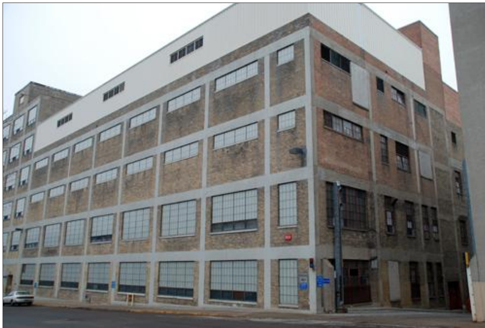
FIGURE 8. BUILDING 14, FAÇADE AND EAST ELEVATION, FACING NORTHWEST
