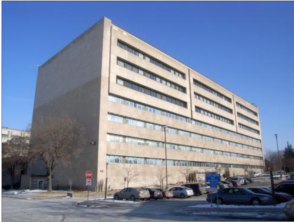
FIGURE 20. BUILDING 42, FAÇADE, FACING NORTHEAST
