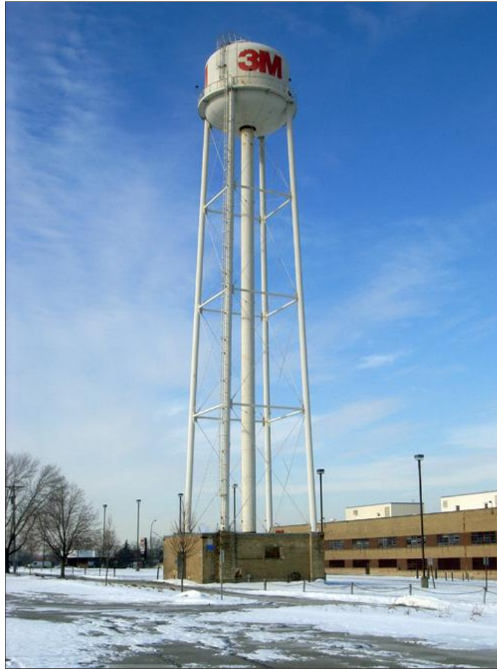
FIGURE 18. BUILDING 40, 3M WATER TOWER AND PUMP HOUSE, FACING NORTHWEST
