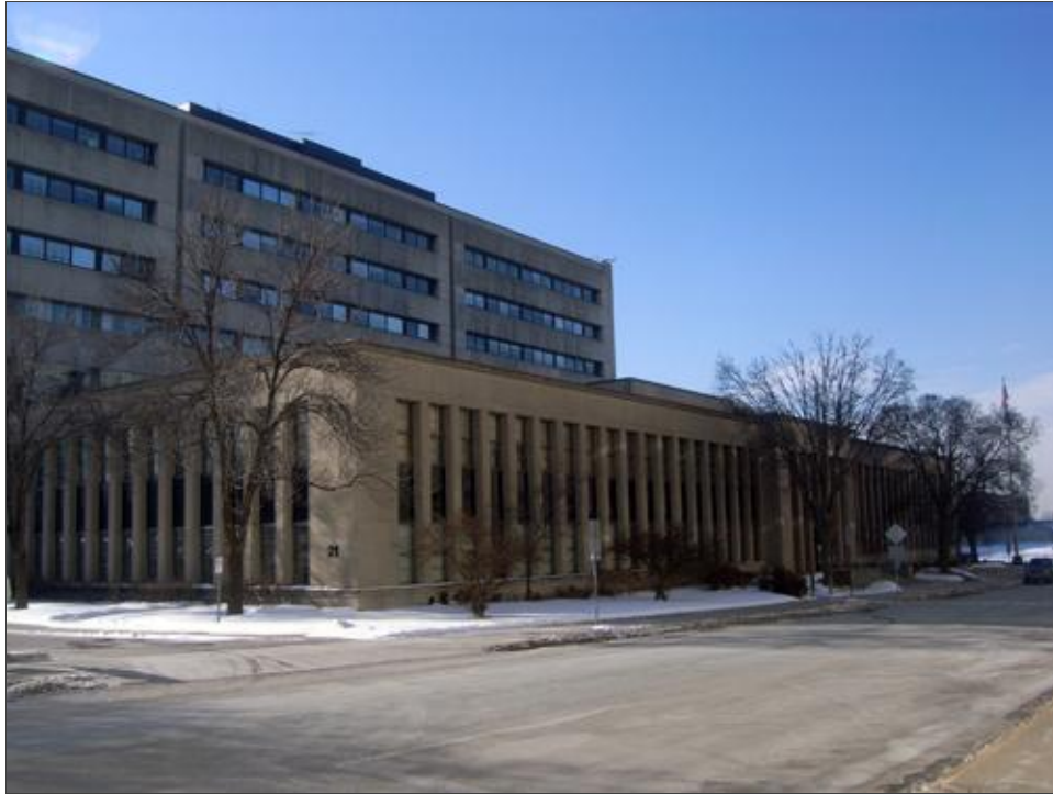
FIGURE 11. BUILDING 21, FAÇADE, FACING SOUTHWEST
