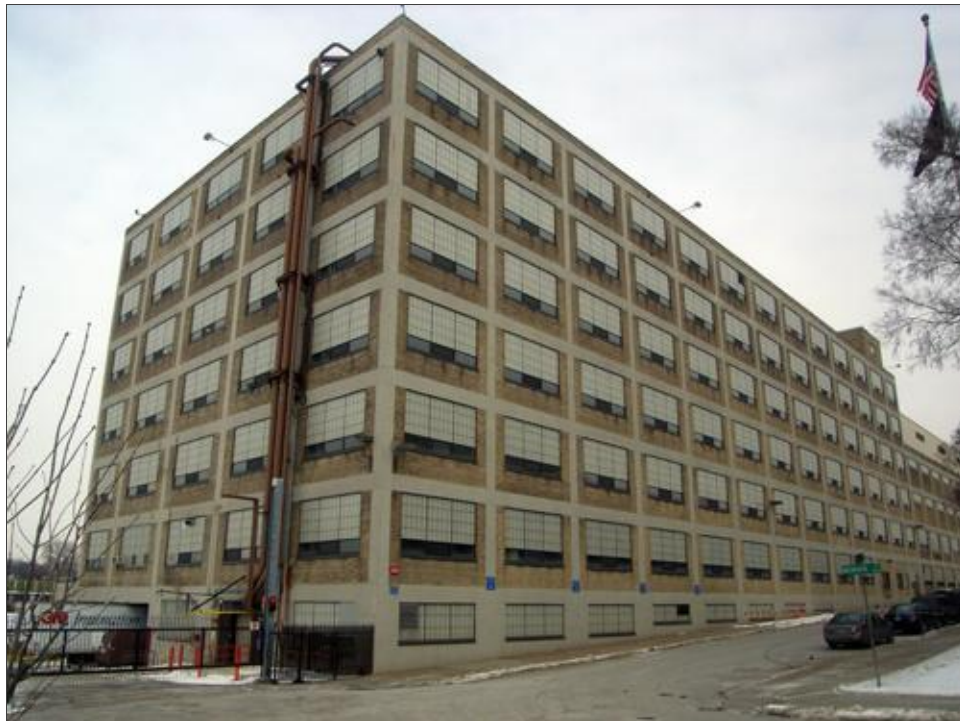
FIGURE 9. BUILDING 20, SOUTH AND WEST ELEVATIONS, FACING NORTHEAST
