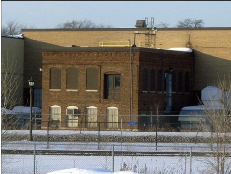
FIGURE 23. BUILDING 80, FAÇADE AND EAST ELEVATION, FACING NORTHWEST
