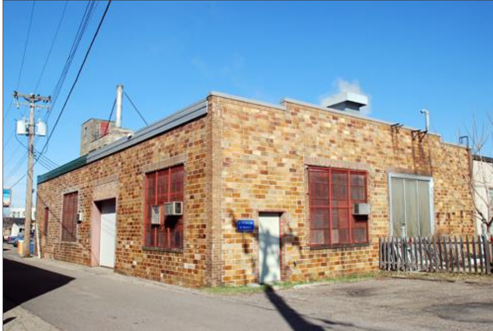
FIGURE 16. BUILDING 28, EAST AND SOUTH ELEVATIONS, FACING NORTHWEST
