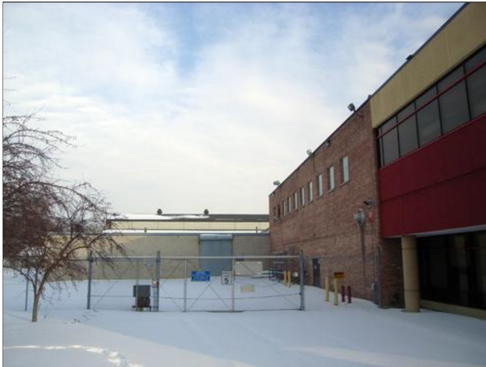
FIGURE 28. BUILDING 91 (BUILDING 99 IN FOREGROUND), NORTH ELEVATION, FACING EAST
