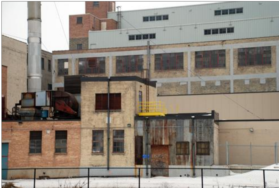
FIGURE 7. BUILDING 45, FAÇADE, FACING SOUTH
