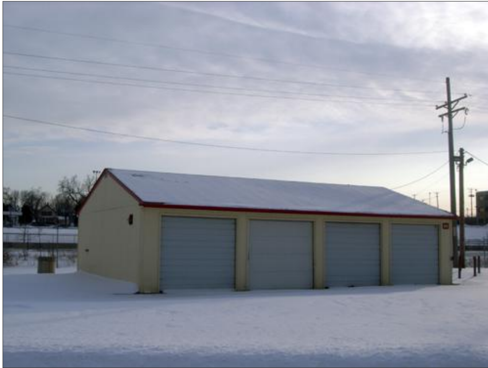
FIGURE 21. BUILDING 84, FAÇADE, FACING SOUTHWEST
