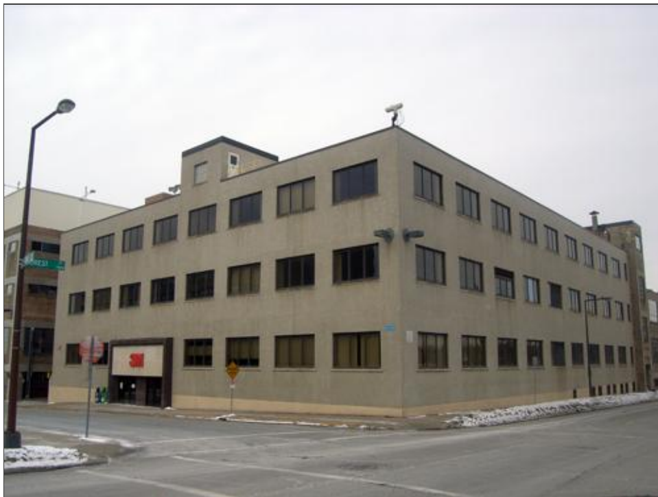
FIGURE 4. BUILDING 2, FAÇADE AND EAST ELEVATION, FACING NORTHWEST
