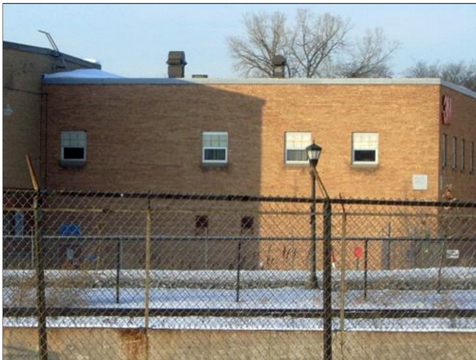
FIGURE 27. BUILDING 98, SOUTH ELEVATION, FACING NORTH
